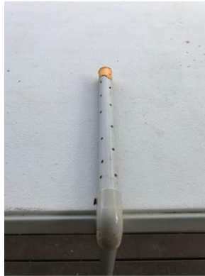
Photo 2– Spreader pipe- underneath view
